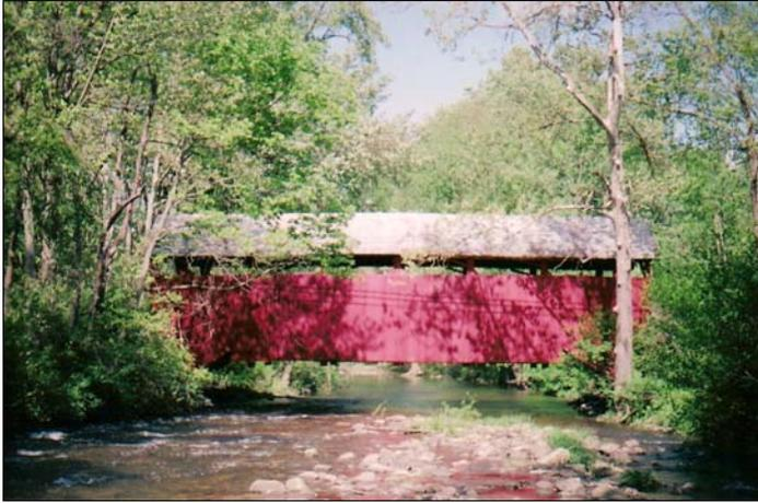
The Factory Bridge, also called the Horsham Bridge, is 60 feet long. Built in 1890, it crosses White Deer Creek near the town of White Deer. Reinforced I beams have been placed under its decking to allow the bridge to support much heavier loads.
