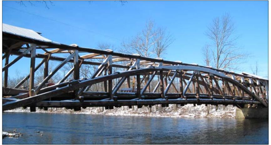
Shown above is a view of the Millmont Covered Bridge taken December 20, 2009 during the time it was undergoing major renovations. Many of the original timbers used in the construction of this bridge were replaced during this process. Below is a view of the Glen Iron Covered Bridge prior to being demolished in June 1952.
